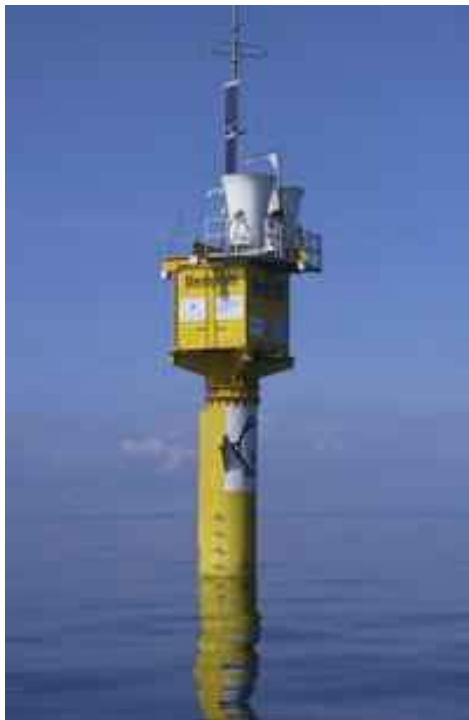
picture 3: measuring mast SKY2000
