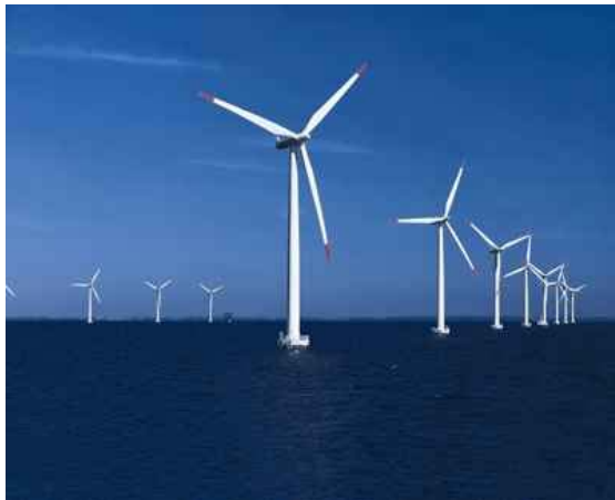
picture 6: wind energy constructions at Baltic I
