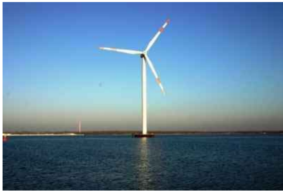
picture 4: wind power construction Breitling
